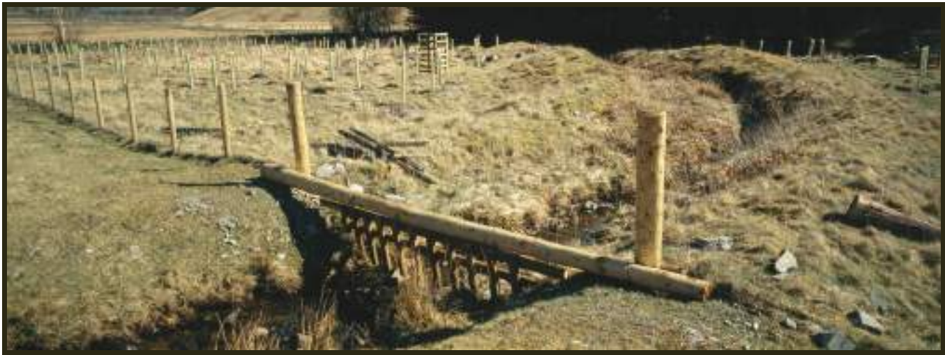
Fig. 7: A well-designed hinged water barrier straddling an upland stream, which prevents deer and livestock access while allowing debris to pass through.
