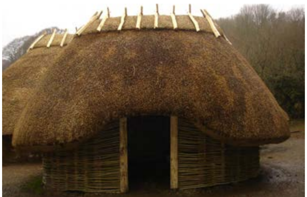
A replica of a Viking dwelling at the Irish National Heritage Park, Ferrycarrig, Co. Wexford, based on dimensions from archaeological digs in Dublin and Wexford. The dwelling was constructed by Muintir na Coille during 2012 and 2013, using small diameter material sourced from native woodlands. (Photo J. Gowran)
